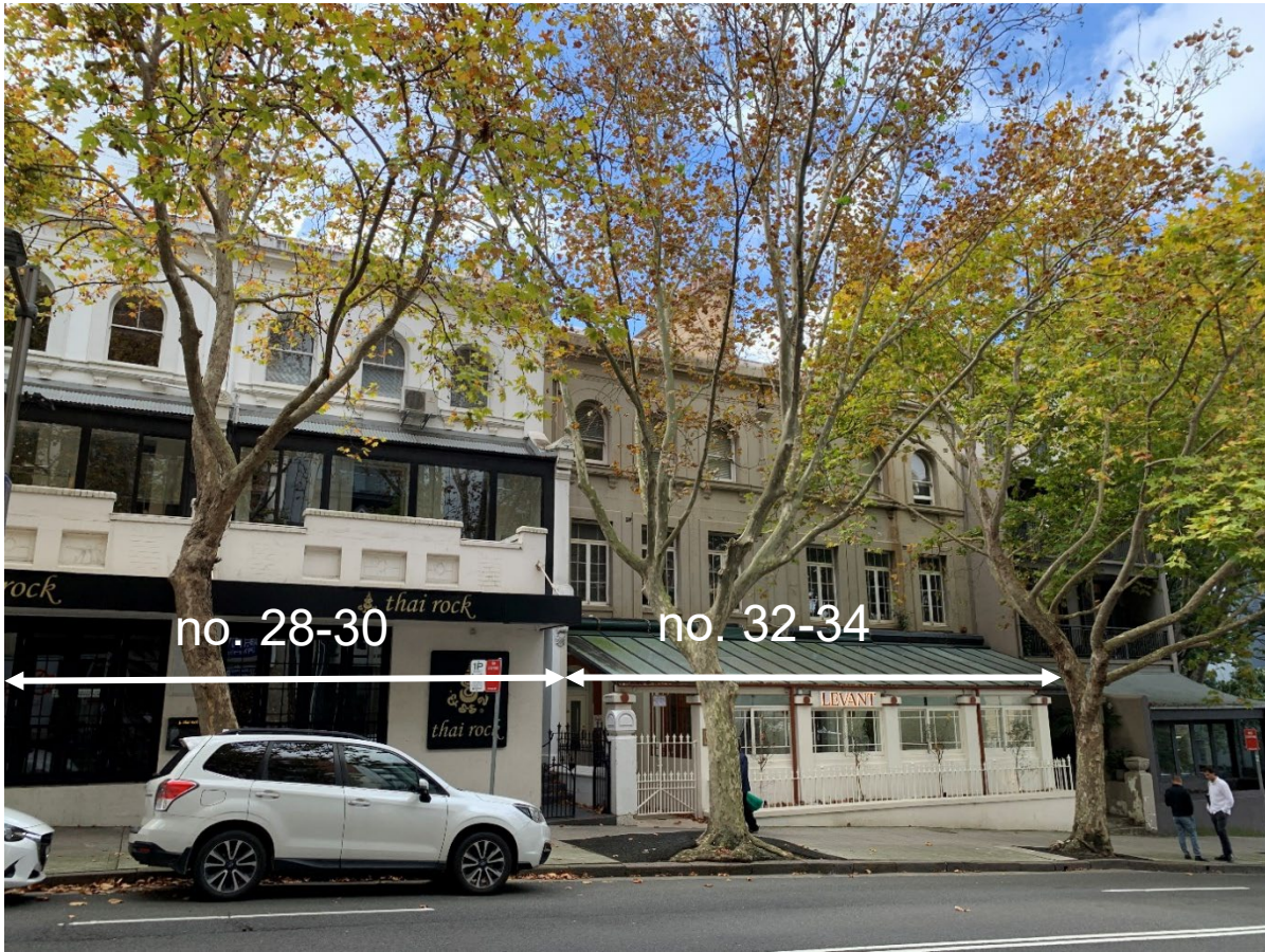
part of site (no. 28-34) viewed from Bayswater Road
