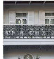
Z - INDICATIVE RECONSTRUCTED CAST IRON BALUSTRADE
