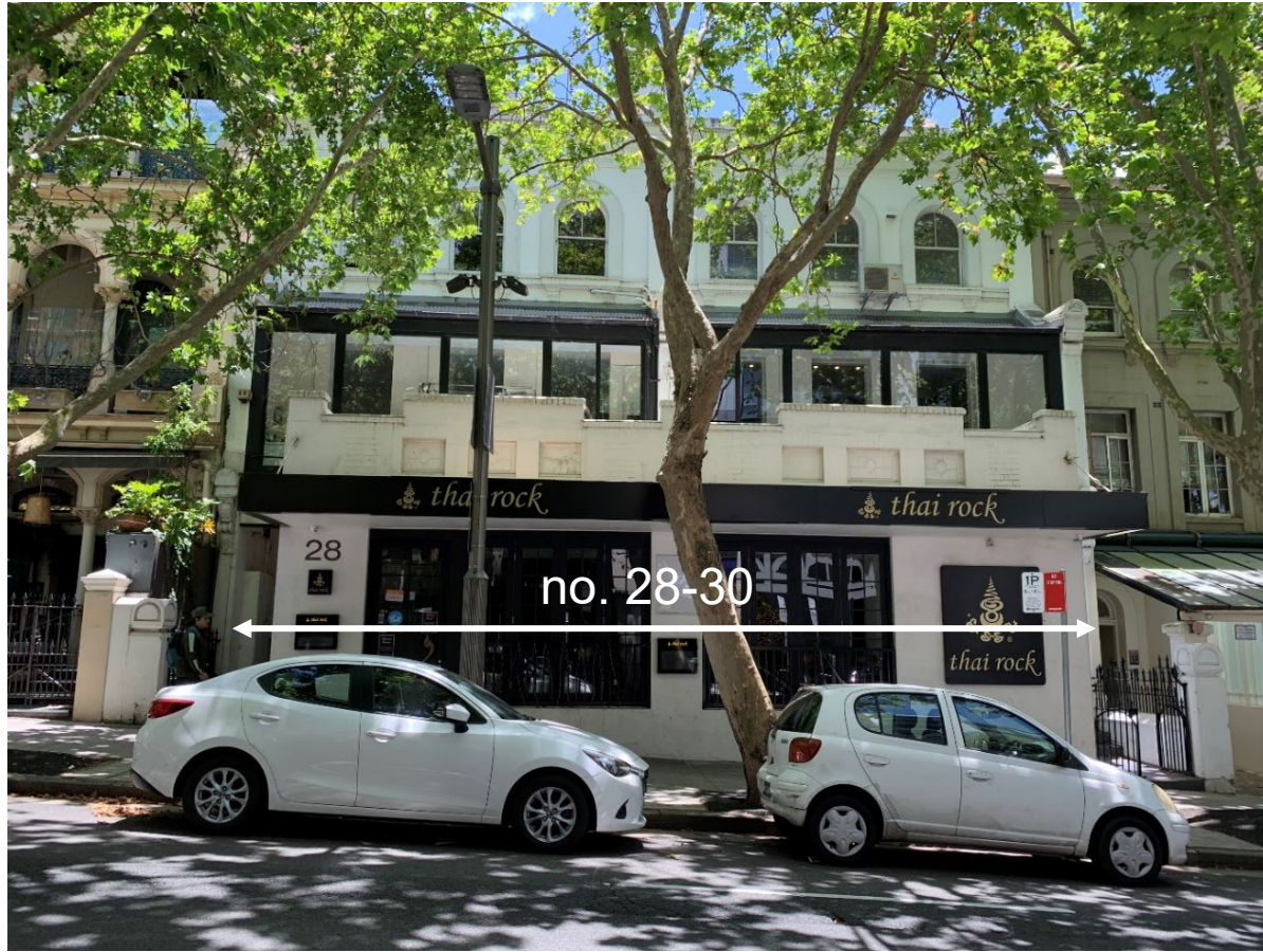
part of site (no. 28-30) viewed from Bayswater Road
